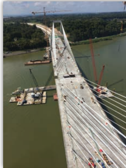
Walsh-Vinci JV on the Ohio River Bridge East End Crossing installing the last pre-cast sections of the cable stay bridge.
