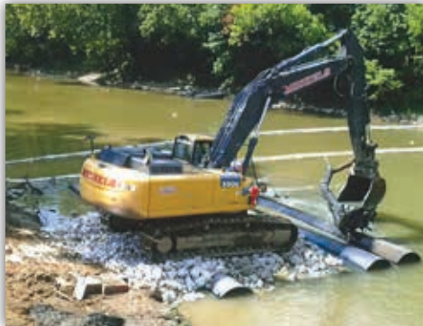
Michaels Pipeline at the Licking River crossing in Nicholas County.
