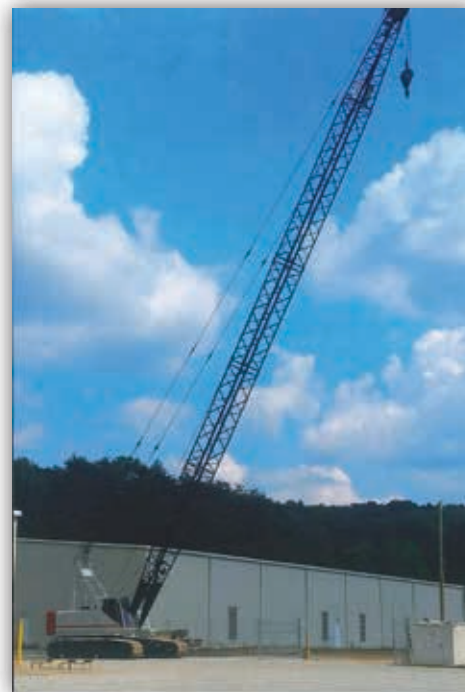
Link-Belt Crawler Crane at the Boston Training Site.
